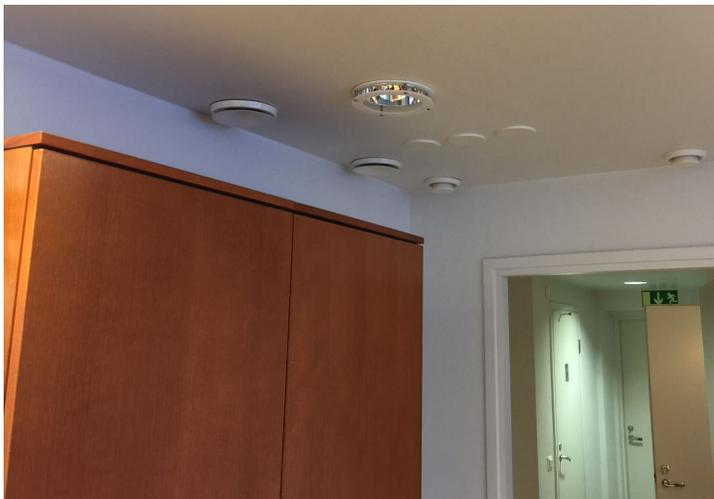
Negotiation room had plenty of terminal devices, but ventilation is still insufficient. During measurement period, CO<sub>2</sub> levels reached measurement equipment's maximum values of 2000 ppm, which is clearly over all guidelines.
