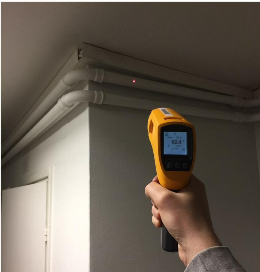
Picture 2: Non-insulated heat pipe in corridor 103.
