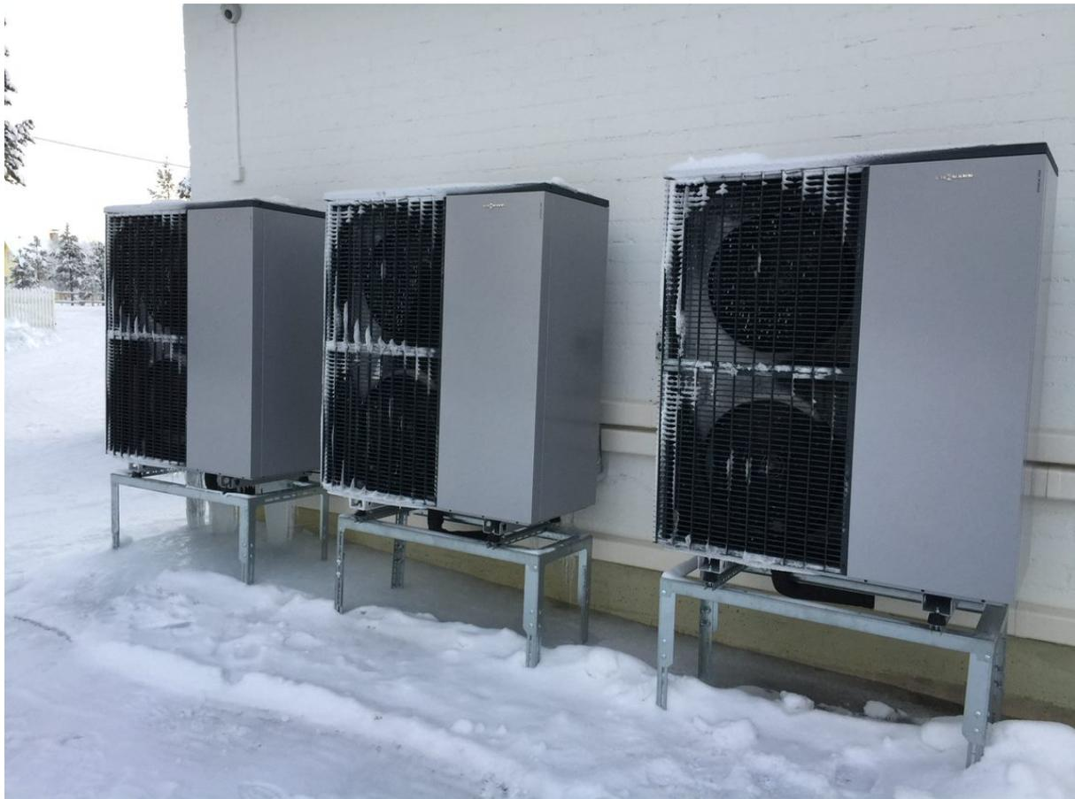
Figure 1: Outdoor units of the heat pumps
