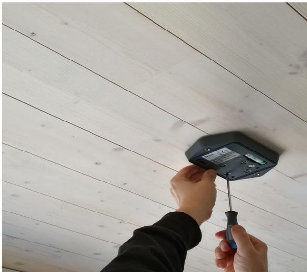
Picture 3. Fixing the sensor directly onto the CLT in the DAS Kelo building, Pirttinen Valterri LaplandUAS:
